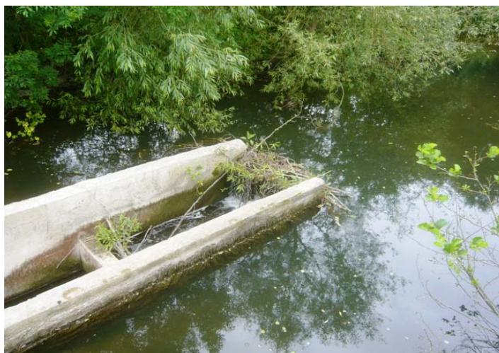
Holgate weir before modification
