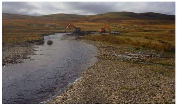
Extraction taking place October 2018. WUF staff using plant to scrape back dry gravel ready to be loaded onto lorries
